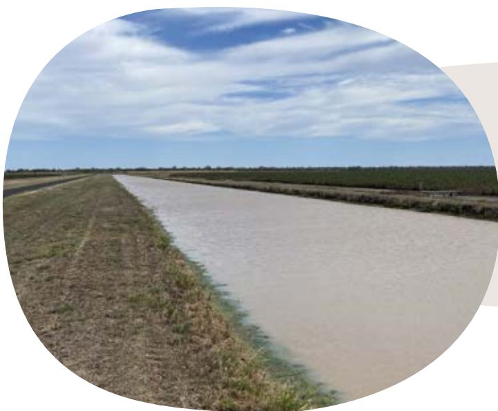
Irrigation supply channel, St George, QLD.
